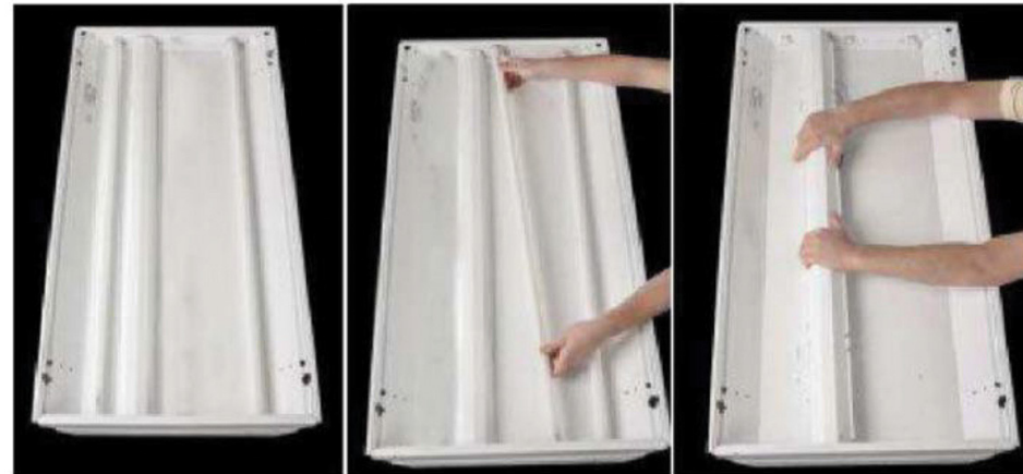
A. REMOVE TROFFER LENS TO EXPOSE LAMPS AND BALLST COVER
